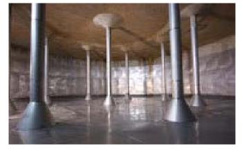
Stainless steel linings of concrete reservoirs. Source: www.forstenlechner.at
