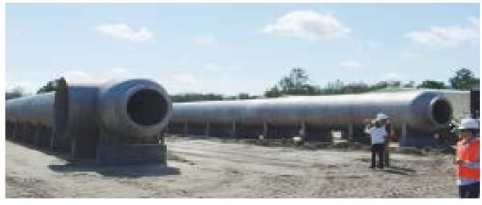
Picture above: Pipework for the hydrogen sulphide removal stage of waterworks. Source: Dixie-Southern Duelle, Fla (USA), www.thefabricator.com Pictures below: Type 316 stainless steel for the City of Lake Worth reverse osmosis water treatment plant. Source: Mock & Roos (USA), www.mockroos.com
