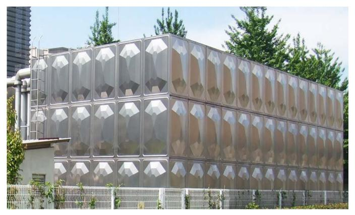
Modular water tank system made from stiffened stainless steel panels. Photo: Morimatsu (Japan), www.morimatsu.co.jp
